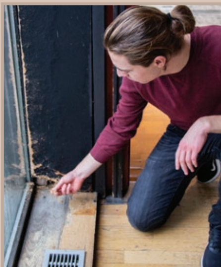
UKEleader Jørgen Bonden and AU leader Jens Bartnes is showing the worn-out windows creating the loss of heat.
